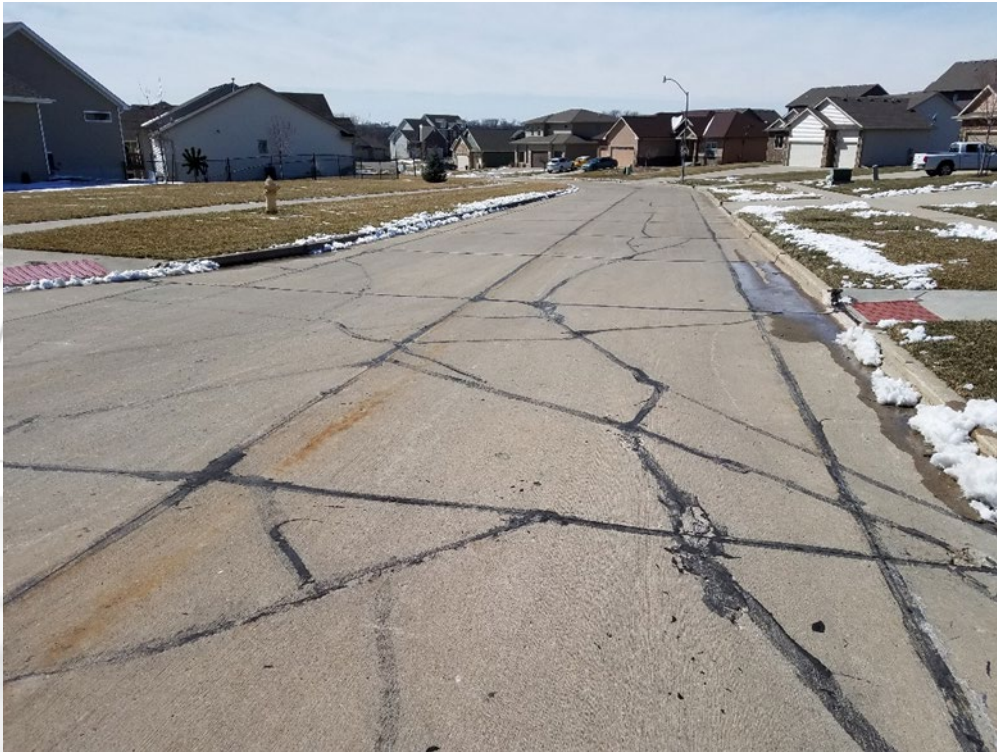
12-Year Pavement - Current
