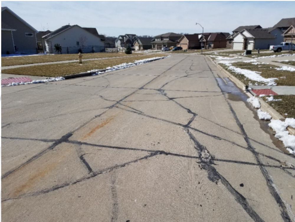
12-Year Pavement - Current
