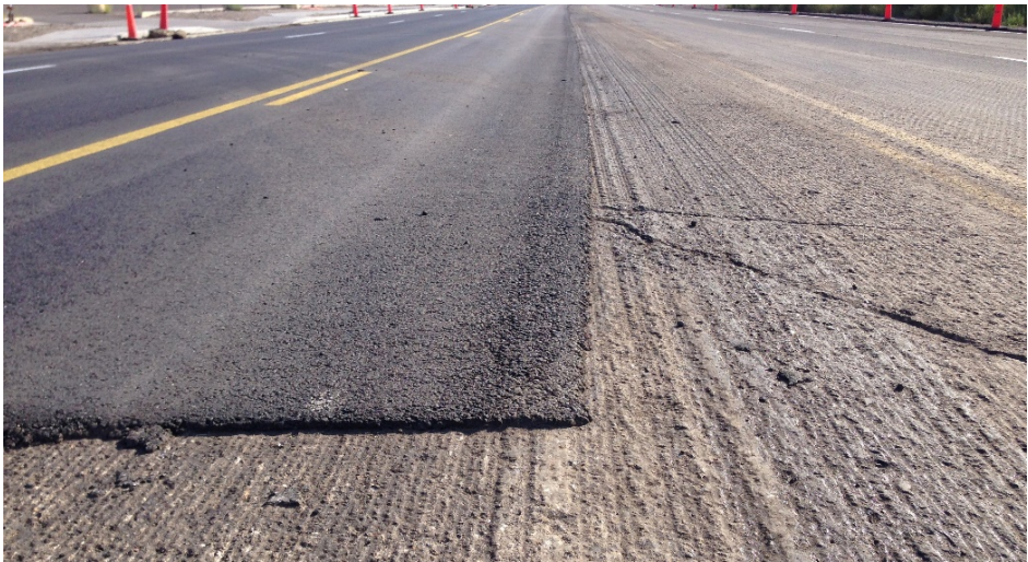
FIGURE 28: HMA OVERLAY PLACED ON MILLED PAVEMENT (FAMARTIN)
