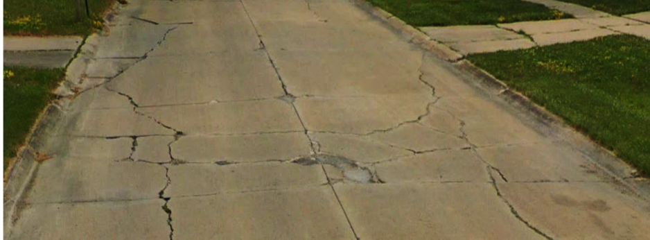
FIGURE 19: EXAMPLE OF “POOR” CONDITION (PCC) – 11TH STREET SE This image shows a PCC street whose pavement is rated 25/100 and considered “Poor” due to a large number of failures and cracking.
