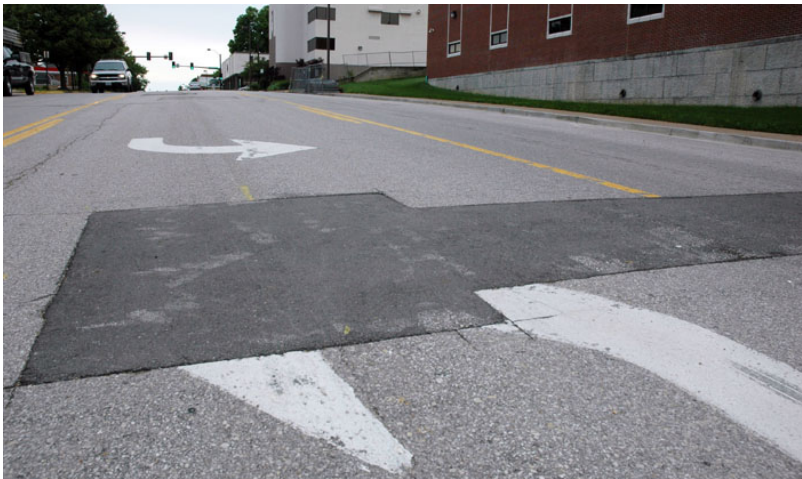
FIGURE 33: HMA PATCHING WITH LOCALIZED PAVEMENT REMOVAL (KOMU) This is an example of an asphalt patch applied with appropriate localized removals and some base repair.
