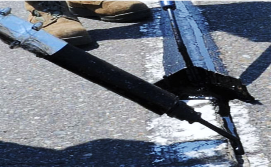
FIGURE 30: CRACK SEALING PERFORMED W/ ROUTING (USAF/KENNA JACKSON) This is an example of crack sealing being performed with special preparation in the form of using a router to clean up the crack profile, as being performed by 35th Civil Engineer Squadron.
