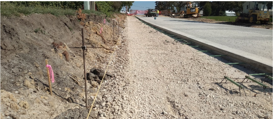
FIGURE 27: RECONSTRUCTION OF DIVISION STREET
