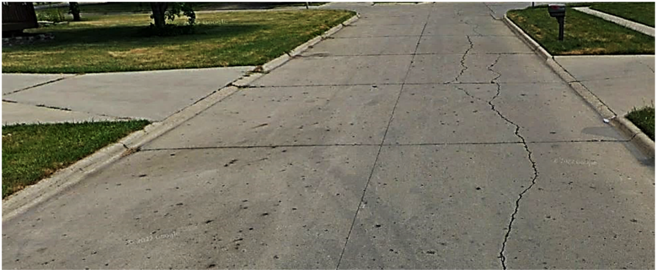
FIGURE 15: EXAMPLE OF “GOOD” CONDITION (PCC) – 5TH STREET SE This image shows an example of a PCC pavement in “Good” condition. 5 th St SE was rated as 73/100, because some roughness and minor cracking.
