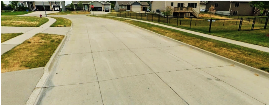
FIGURE 13: EXAMPLE OF “VERY GOOD” CONDITION (PCC) – EVERGREEN DR. This image of Evergreen Dr shows an example of a “Very Good” PCC pavement, and it was rated as a perfect 100/100.
