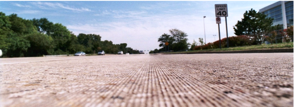
FIGURE 31: PAVEMENT AFTER DIAMOND GRINDING (JOHN ROBERTS). This picture shows the texture of PCC pavement after diamond grinding was used on it. The image was taken on a project near Chicago, Illinois.
