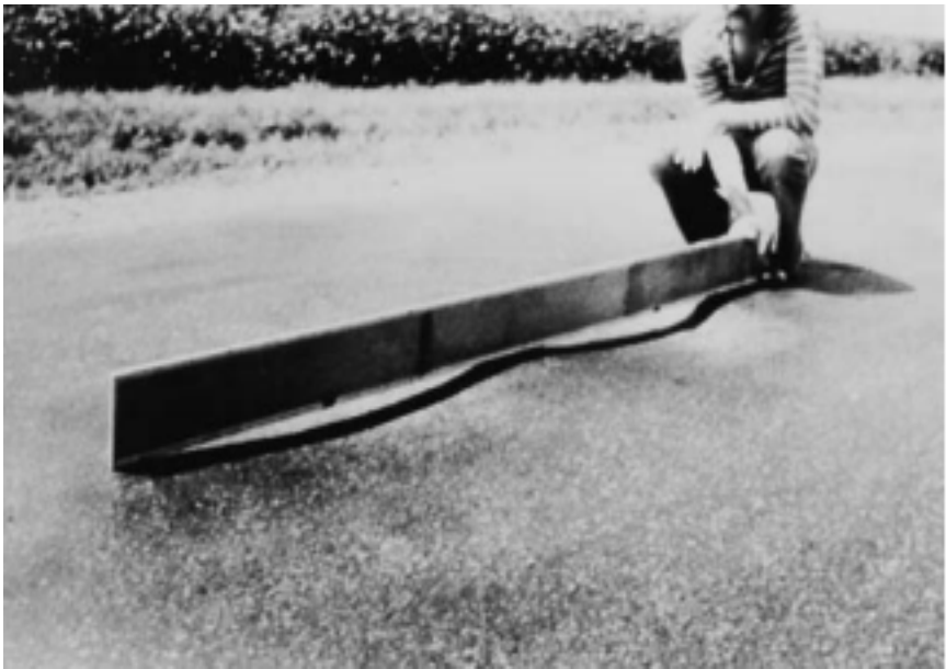
FIGURE 7: EXAMPLE OF DISTORTION (ASTM)
