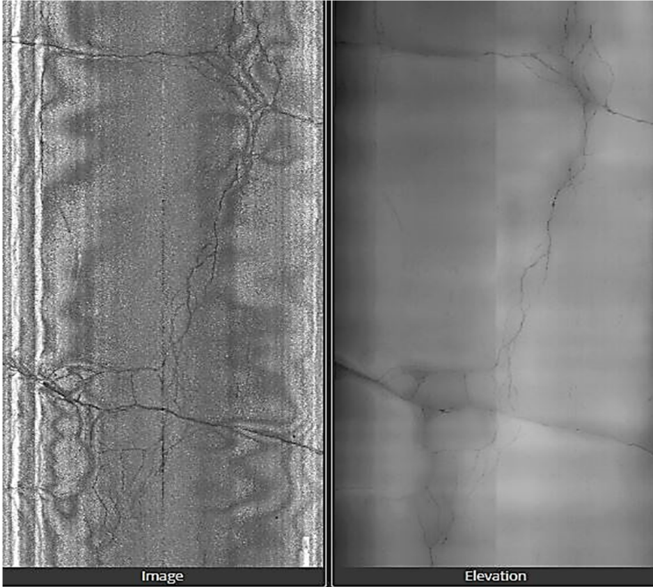
FIGURE 21: ROADWAY IMAGERY OF A “FAIR” ACC PAVEMENT THIS IMAGERY IS FROM THE SECTION OF 2ND STREET SHOWN. THESE WERE CAPTURED BY THE DATA COLLECTION VEHICLE’S DOWNWARD FACING CAMERA (LEFT) AND LIDAR ARRAY (RIGHT). THESE ARE ONE OF THE KEY RESOURCES USED IN EVALUATING PAVEMENT CONDITION.
