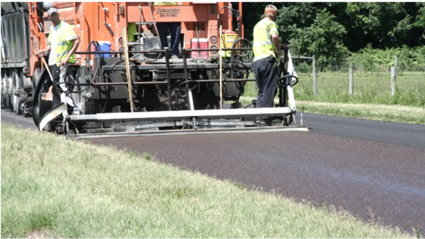
FIGURE 32: MICROSURFACING CREW AT WORK. (ERIC PULLEY). This picture shows a crew using a Microsurfacing machine to lay a new surface on this street.
