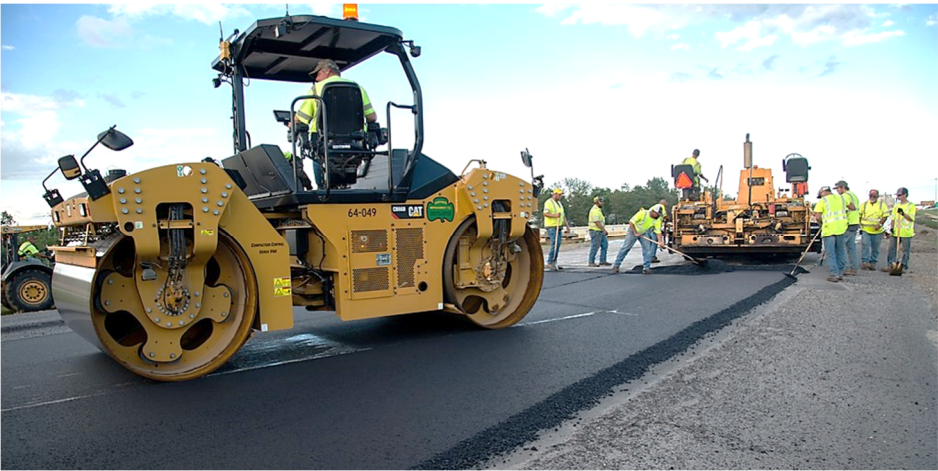
FIGURE 26: RECONSTRUCTION OF I-94 (NDDOT)
