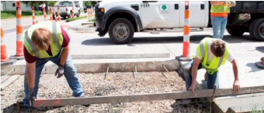
FIGURE 29: PCC RESTORATION (CITY OF CEDAR RAPIDS) This is a picture of a city maintenance crew in Cedar Rapids performing a panel replacement as part of a larger concrete restoration project.
