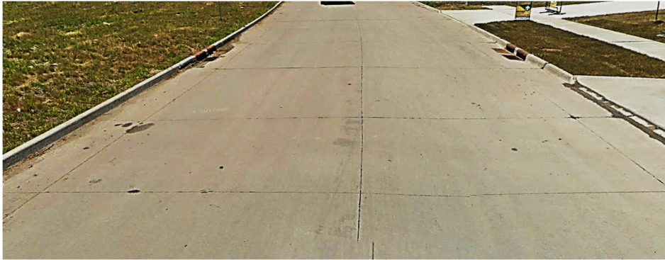
FIGURE 12: EXAMPLE OF “VERY GOOD” CONDITION (PCC) – ALEXANDER DR. This picture of Alexander Drive was rated a very high PCI of 90 /100 because it demonstrates no visible pavement distresses.
