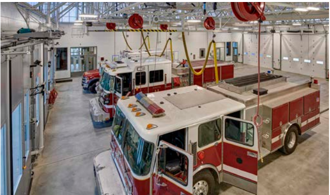
Figure 1.8 Emergency Services Interior Example
