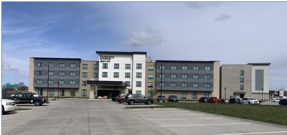
Figure 25 – Fairfield Inn &amp; Suites Altoona
