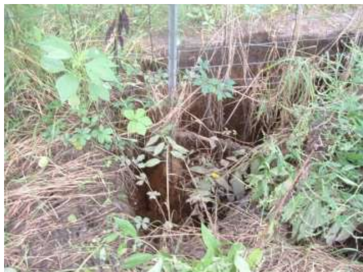
Figure 105. Photo of Sinkhole Near Runnells, July 2010
