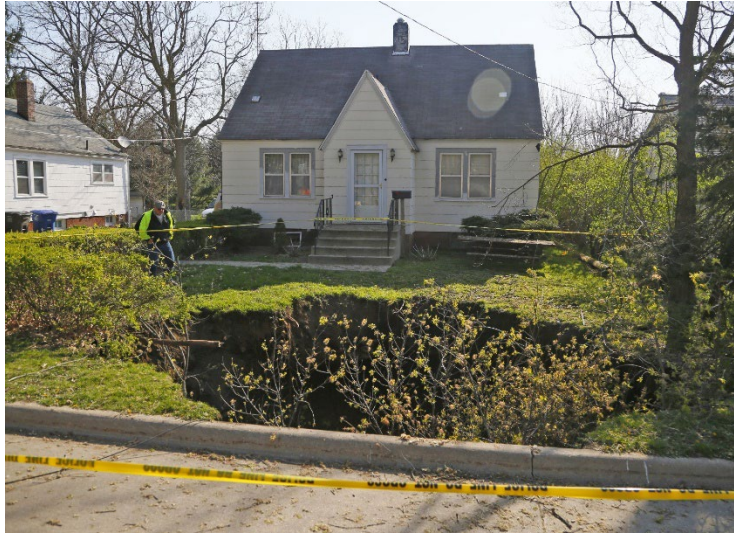
Figure 104. Photo of Sinkhole Near Runnells, July 2010
