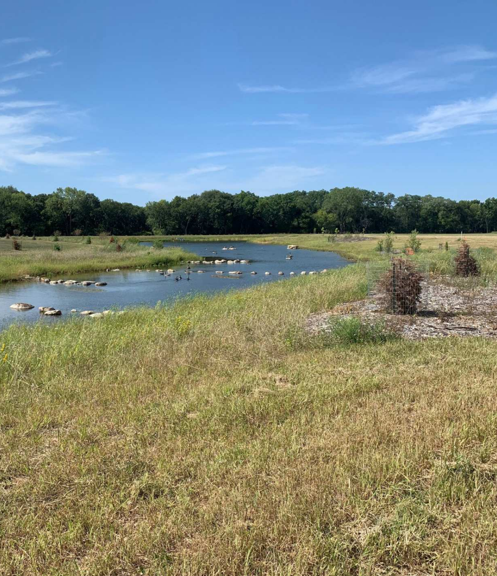
Rock dams made of stones to slow stormwater and allow sediment settling. Image Credit: Polk County Public Works
