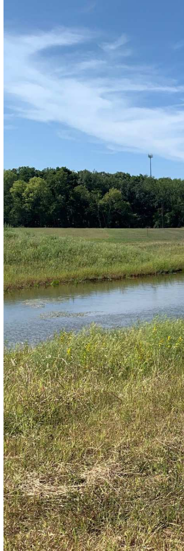
This green infrastructure pond in Pleasant Hill, Iowa, uses che...
