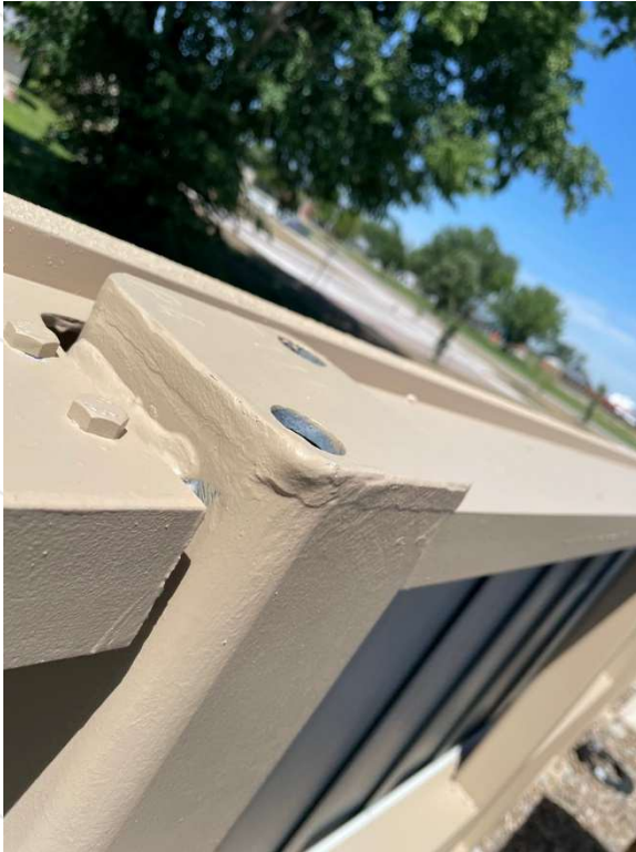
Core Drilled weep holes
