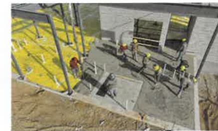
Precast Concrete Installation & Cast-in-Place Concrete
