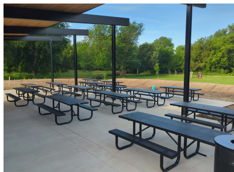
Walker-Johnson Park Shelter Urbandale, Iowa
