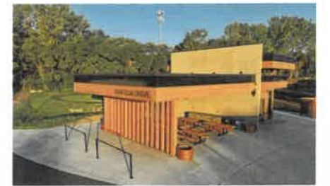
Rough & Finish Carpentry
