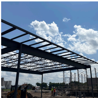
Structural Steel Erection
