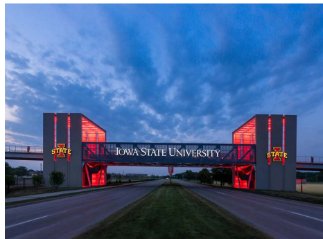
ISU Jack Trice Stadium Pedestrian Bridge Ames, Iowa
