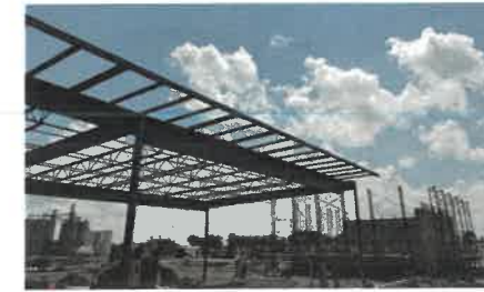
Structural Steel Erection
