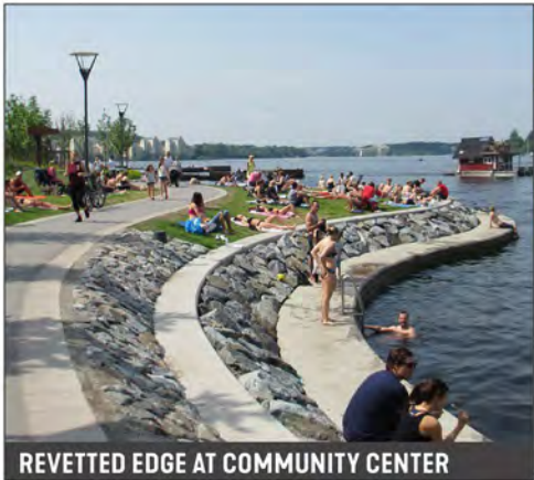
REVETTED EDGE AT COMMUNITY CENTER
