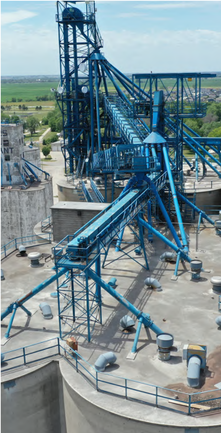
Grain Elevator Deck 2022 Drone Deploy
