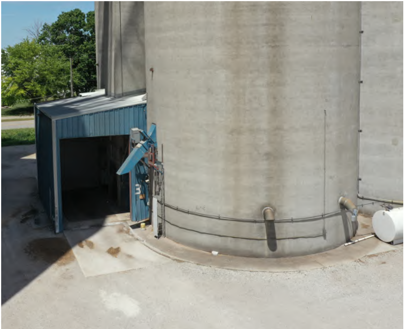
Receiving Enclosure 2022 Drone Deploy
