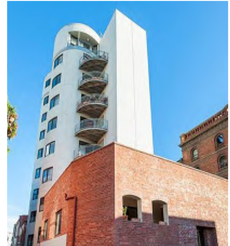
Victoria Distillery + Silos Collingwood, Australia
