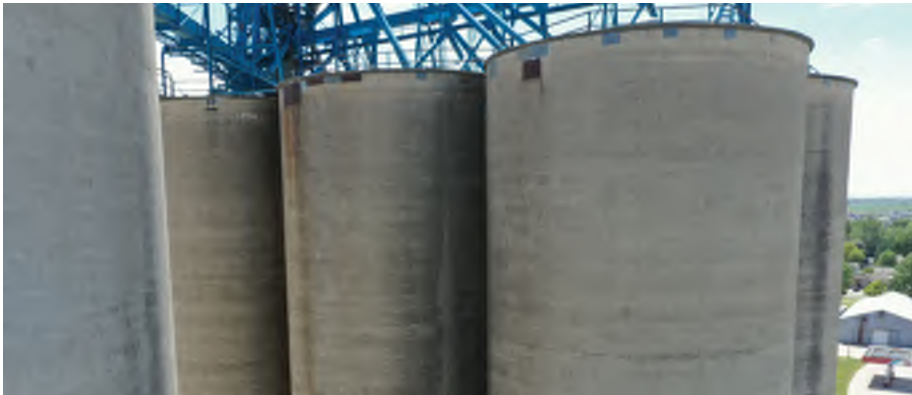
Cast Concrete Walls
