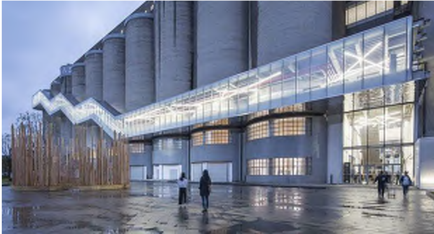
Minsheng Wharf Atelier Liu Yuyang Architects 2018 Shanghai, China
