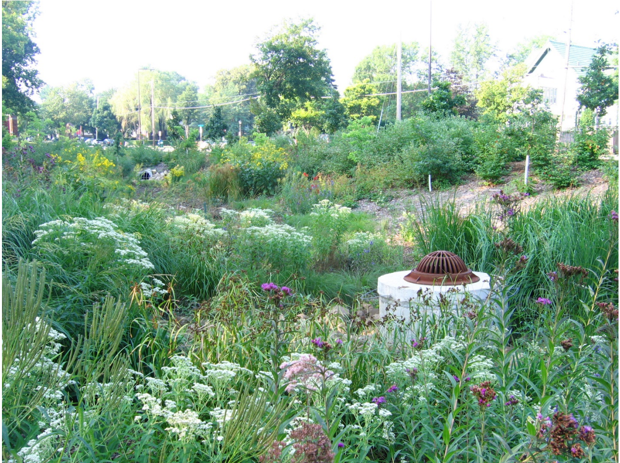
Figure 29. Bioretention cell example.
