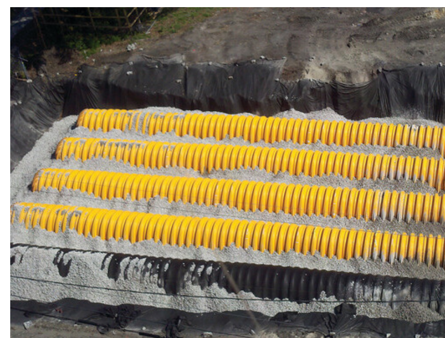
4 STORMWATER UNDERGROUND STORAGE
