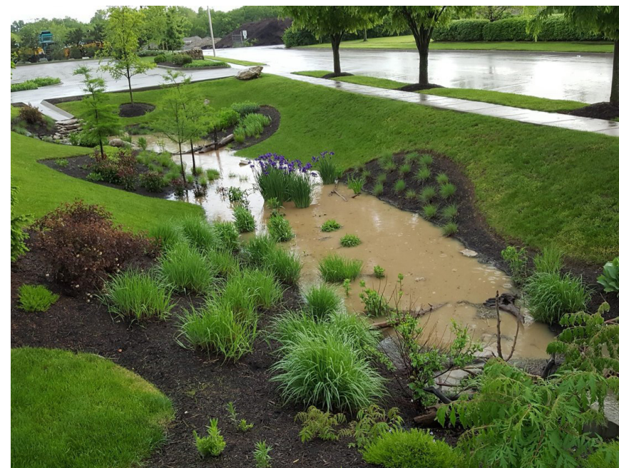
1 RESIDENTIAL STORMWATER DETENTION
