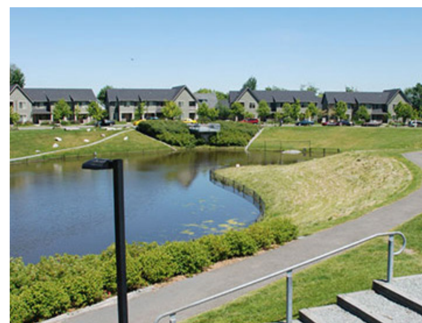
6 STORMWATER RETENTION POND
