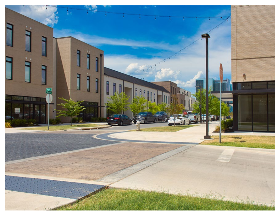
1 RAISED PEDESTRIAN CROSSING
