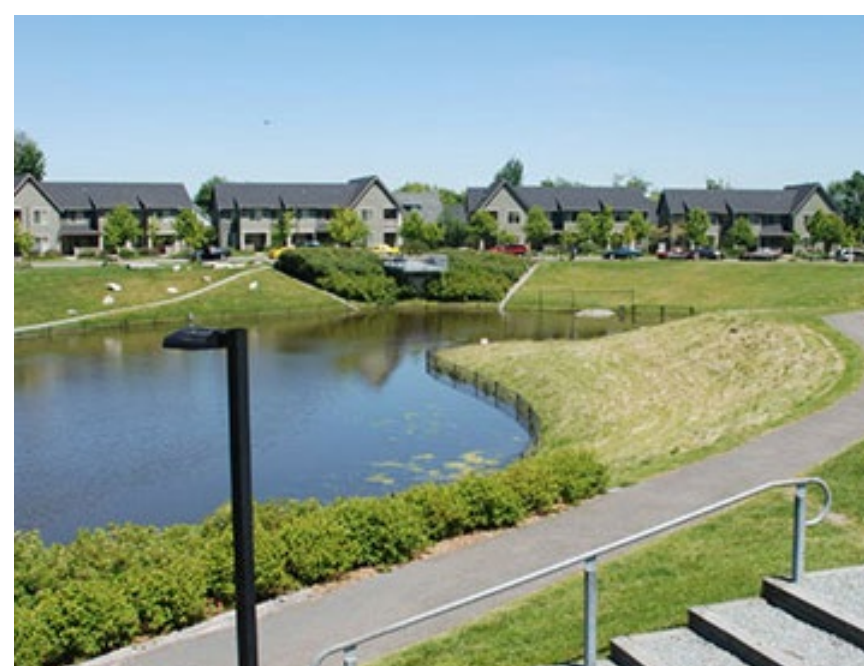
6 STORMWATER RETENTION POND
